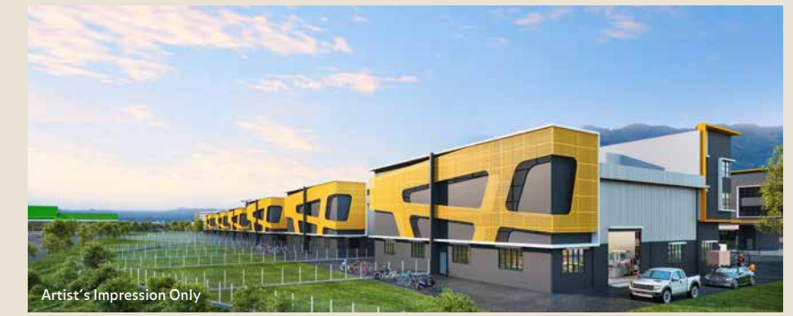
Rear View (Facing Nilai Impian Toll Plaza)
