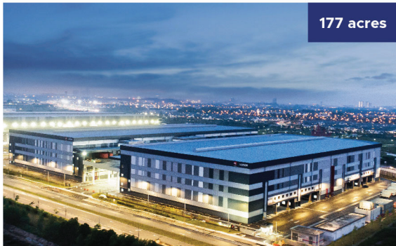
E-Metro Logistic Park
