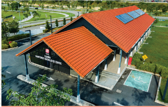
The Elmina Rainforest Knowledge Centre (“ERKC”) earns accolades in the “Environmental Category” at the FIABCI Malaysia Property Award 2023
